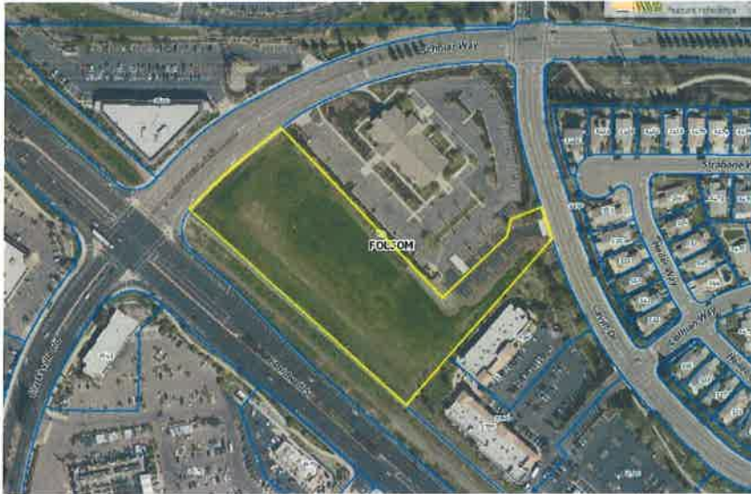
FIGURE 1: SAGE PROJECT SITE- AERIAL PHOTOGRAPH
